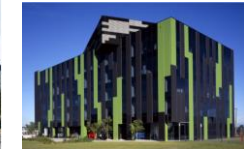
Innovation Building, Melbourne (2)
