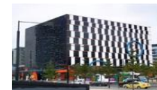
1010 La Trobe Building 1, Melbourne (S$142.5m)
