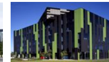
1010 La Trobe Building 2, Melbourne (S$142.5m)
