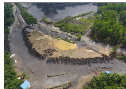
BEFORE - EX-TAILING AREA PRIOR TO REHABILITATION WORKS
