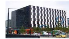
1010 La Trobe Building 1, Melbourne
