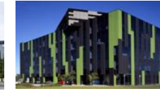
1010 La Trobe Building 2, Melbourne
