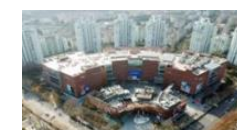
Suntec Place – Sanlin Mall
