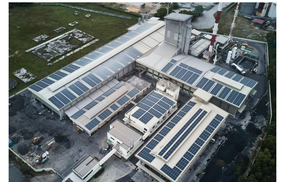
MSC's new smelting facility in Pulau Indah
