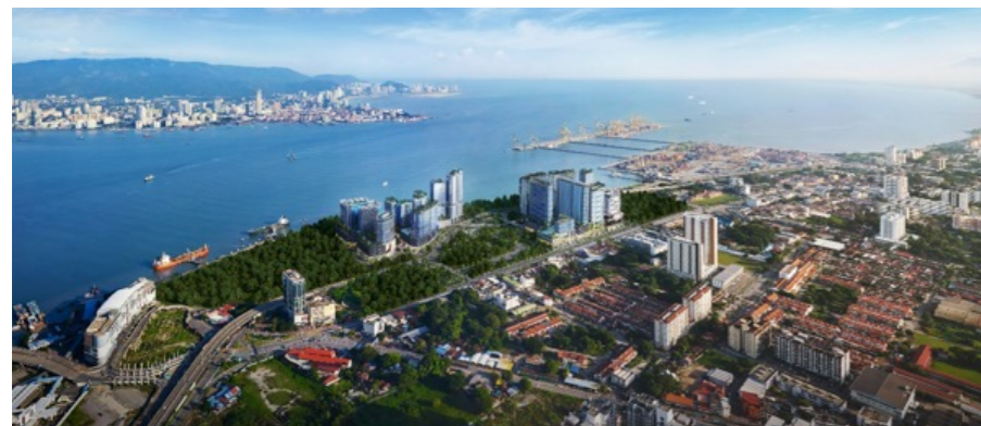
Aerial view of Straits City site
