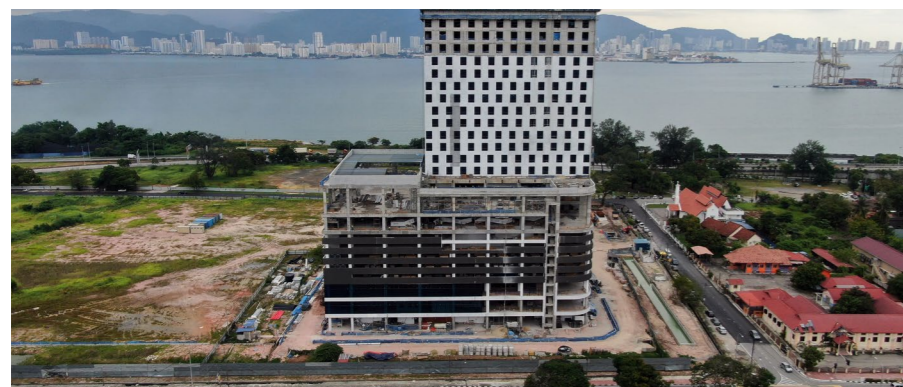
Construction of 4-star hotel in Straits City
