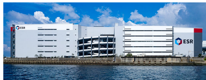
ESR Amagasaki Distribution Centre
